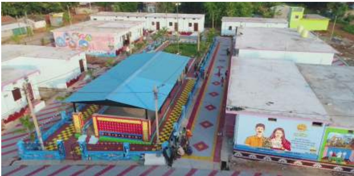
Figure 69. View of the Parichaya Centre
