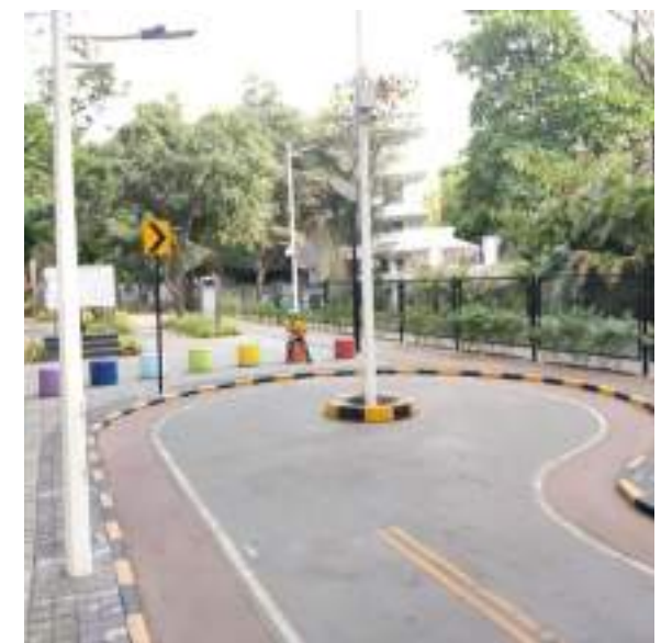
Figure 41. View of traffic park at Aundh road
